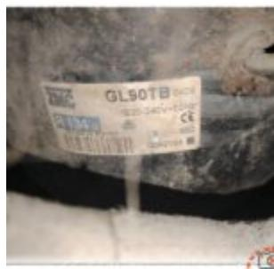
The ZMC GL90TB is a high-performance 1/4 HP compressor designed for High Back Pressure (HBP) commercial refrigeration. Operating on R134a with a 220-240V supply, it offers a cooling capacity of approximately 2800 BTU/h. This article provides technical specs, COP efficiency metrics, and direct replacement models for professional HVAC technicians and industrial cooling experts.
