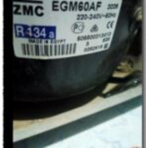
The ZMC EGM60AF is a high-performance hermetic compressor designed for low back pressure applications in domestic refrigeration. Engineered with precision in Egypt, this 1/6 HP unit operates on R134a refrigerant and is tailored for 220-240V 50Hz power systems. It offers a reliable cooling solution for small to medium household refrigerators and upright freezers worldwide.
