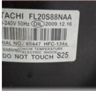
The HITACHI FL20S88NAA 0.75 HP hermetic scroll compressor delivers 256W cooling capacity at 50Hz, utilizing HFC-134a refrigerant for household refrigerator-freezer applications. This LBP-classified unit operates reliably at 220-240V with RSIR starting method, integrated into Sharp's SJ-PT73R-HS3 model offering 662-liter gross capacity with Hybrid Cooling System and Plasmacluster technology.
