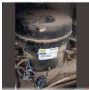
The Konor GPY16AF is a robust hermetic reciprocating compressor engineered for low back pressure applications using R134a refrigerant. With a displacement of 16.2 cm<sup>3</sup>, this 1/2 HP unit is a staple in commercial freezers and large refrigerators. This guide provides detailed technical data, wiring diagrams, and professional cross-reference options for field technicians.
