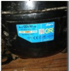
The L55AV and QD59H are cornerstone compressors in the domestic refrigeration industry, both rated at 1/6 HP. While the L55AV traditionally operates with R12, the QD59H is the modern R134a standard. This article provides deep technical data, electrical wiring diagrams, and professional comparison tables for field technicians and refrigeration engineers seeking reliable data.
