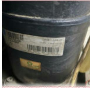
The Tecumseh / L'Unité Hermetique CAJ9480T is a 5/8 HP hermetic compressor delivering about 1 968 W of cooling capacity for R22 commercial refrigeration systems. It is widely used in small cold rooms, display cabinets and compact condensing units. This Mbsmgroup guide explains its main specifications, applications, installation tips and key technical PDFs.
