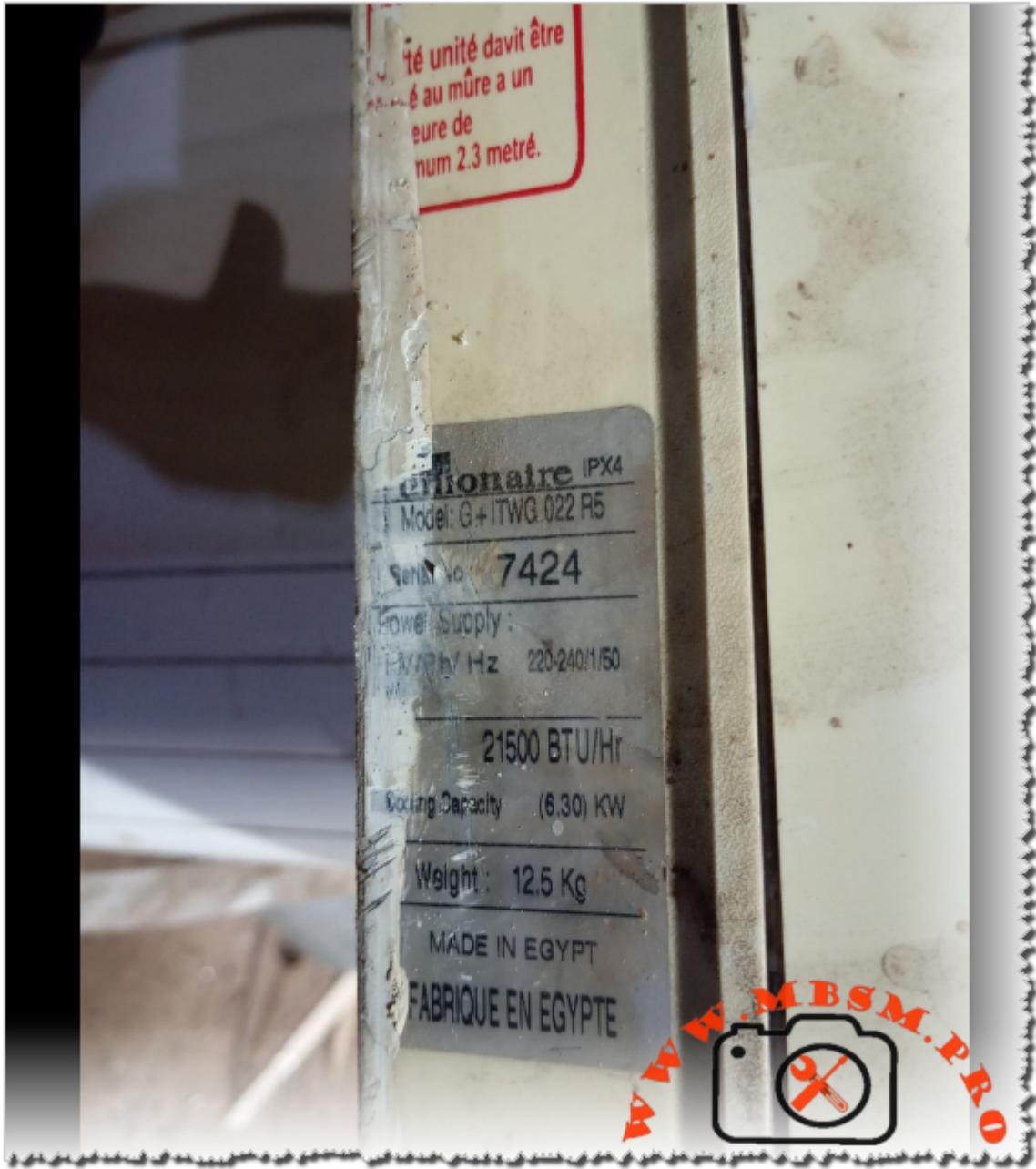
[mbsmpro.com](http://mbsmpro.com)-Unionaire G ITWG 022 R5 Air Conditioner Specifications 21500 BTU Cooling Capacity Technical Manual and Download
