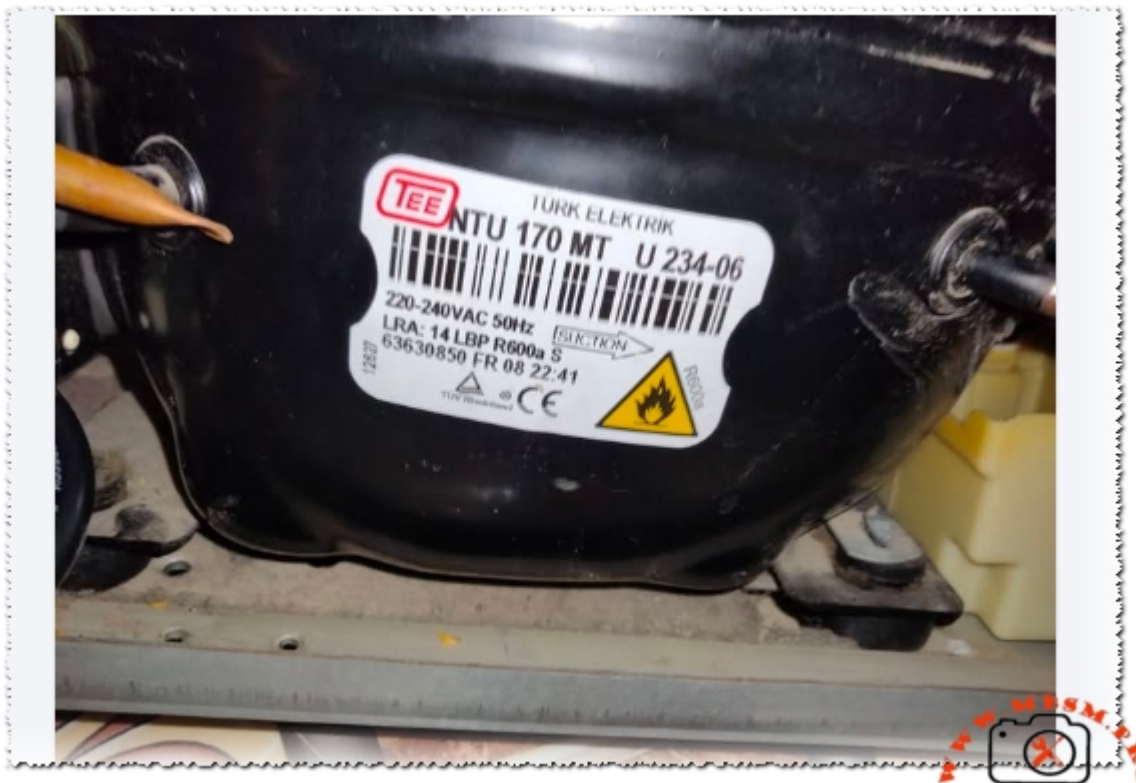
TEE NTU 170 MT Compressor 1/4 HP R600a mbsmpro mpdf (2)Download
