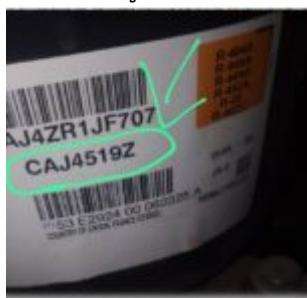
Regarding the compressor in the photo (**Tecumseh CAJ4519Z**) used in a cold room (chilling/positive temperature) with **R-407C** gas, finding frost on the suction line and the expansion valve is **not normal** for this type of application.
