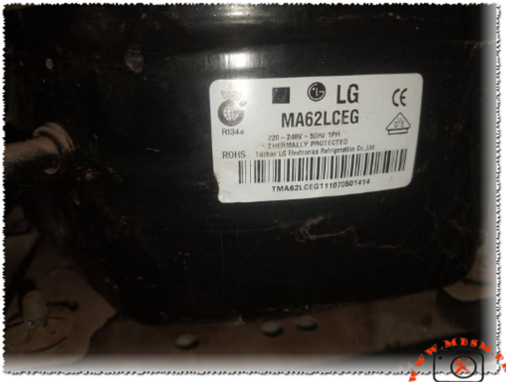
LG MA62LCEG compressor specifications R134a 1/5 hp LBP mbsmpro
