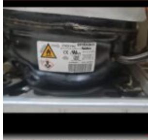
Mbsmpro.com, Compressor, FMXY9C, Embraco, R600a, 1/6 hp, Cooling, 220-240V, 1Ph 50Hz, LBP, Fullmotion, Inverter, -35°C to -10°C, CE UL, Austria
