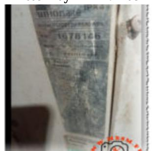
The Unionaire PUQ012HR5R0WPK is a robust 12,000 BTU reversible heat pump system designed for demanding climates. Utilizing an R22 rotary compressor, this unit balances efficiency and reliability. Our technical breakdown covers electrical parameters, pressure ratings, and compatible replacements, providing field workers with the essential data needed for professional maintenance, system repairs, and component sourcing.
