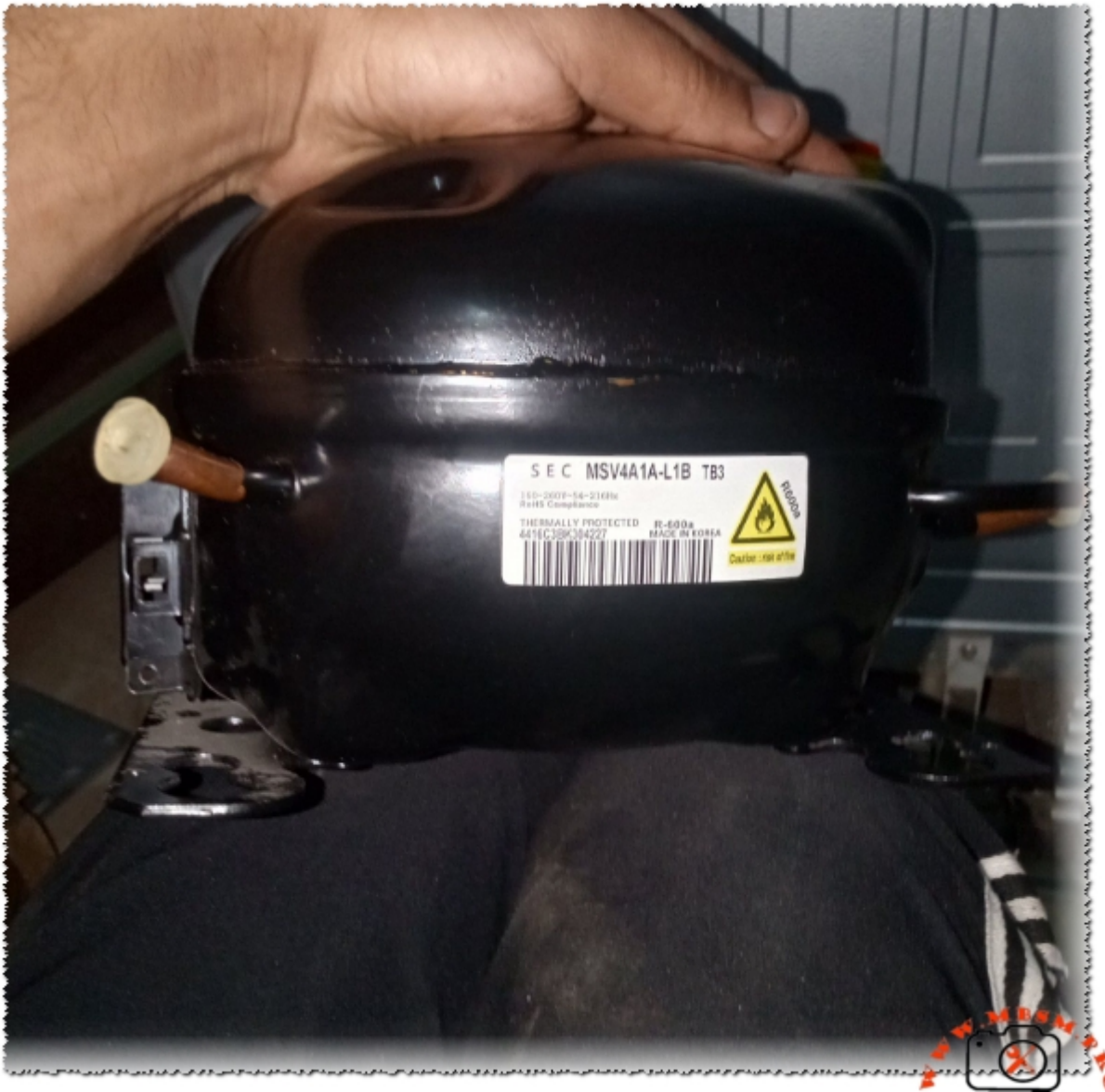
Samsung Compressor, MSV4A1A-L1B, 1/4 hp, Inverter, R600a, 160-260V, 54-216Hz, LBP, BLDC, Cooling/Freezing mbsmpro SAMSUNG-Compressor-Catalogue-2018Download
