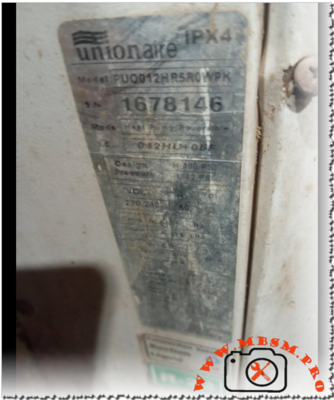
12000 BTU, 2K22S225, ASD102RK, Heat Pump, HVAC, mbsm, mbsm.pro, mbsmgroup, mbsmpro.com, PA145X2C-4FT, PH215X2C-4FT1, PUQ012HR5R0WPK, R22, Rotary Compressor, Unionaire
