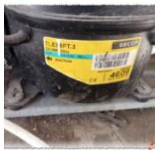
The Secop TLES6FT.3 is a cornerstone of modern domestic refrigeration. This 1/5 HP, R134a compressor is engineered in Slovakia for Low Back Pressure applications, offering a cooling capacity of 149W. Known for its quiet operation and energy efficiency, it is the ideal choice for medium-sized refrigerators and deep freezers looking for long-term reliability.
