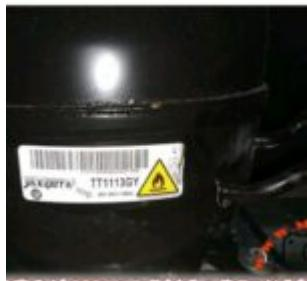
**Mbsmpro.com, Compressor, Jaxipera, TT1113GY, 1/5 hp, Cooling, R600a, 183 W, 1Ph, 220-240V 50Hz, LBP, RSCR/RSIR, -35°C to -15°C, cooling or freezing**
