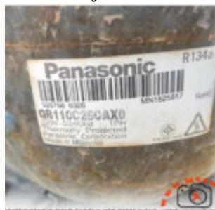
The Panasonic QB110C25CAX0 is a high-performance 1/3 HP reciprocating compressor designed for Low Back Pressure (LBP) applications. Operating on R134a refrigerant, it delivers 280W of cooling capacity at -23.3°C, making it ideal for large domestic freezers and commercial coolers. This guide provides technical data, COP efficiency tables, and compatible replacement models for technicians.
