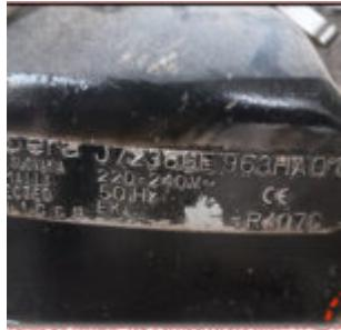
The Aspera J7238GE is a powerhouse in the commercial cooling sector. Delivering 1.5 HP of performance using R407C refrigerant, this Slovakia-built compressor is designed for High Back Pressure applications. With a 32.7 cc displacement and a robust CSR motor, it provides reliable cooling for large-scale industrial chillers and commercial walk-in refrigeration systems worldwide.
