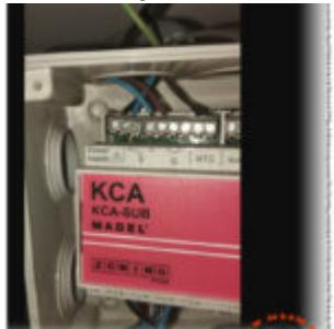
The MADEL KCA-SUB is an electronic zoning controller designed to manage up to six independent air-conditioning zones from a single ducted unit. The image shows the KCA-SUB installed in a junction box with its power, relay and sensor terminals visible, offering HVAC technicians a compact and versatile solution for sub-zone temperature control.
