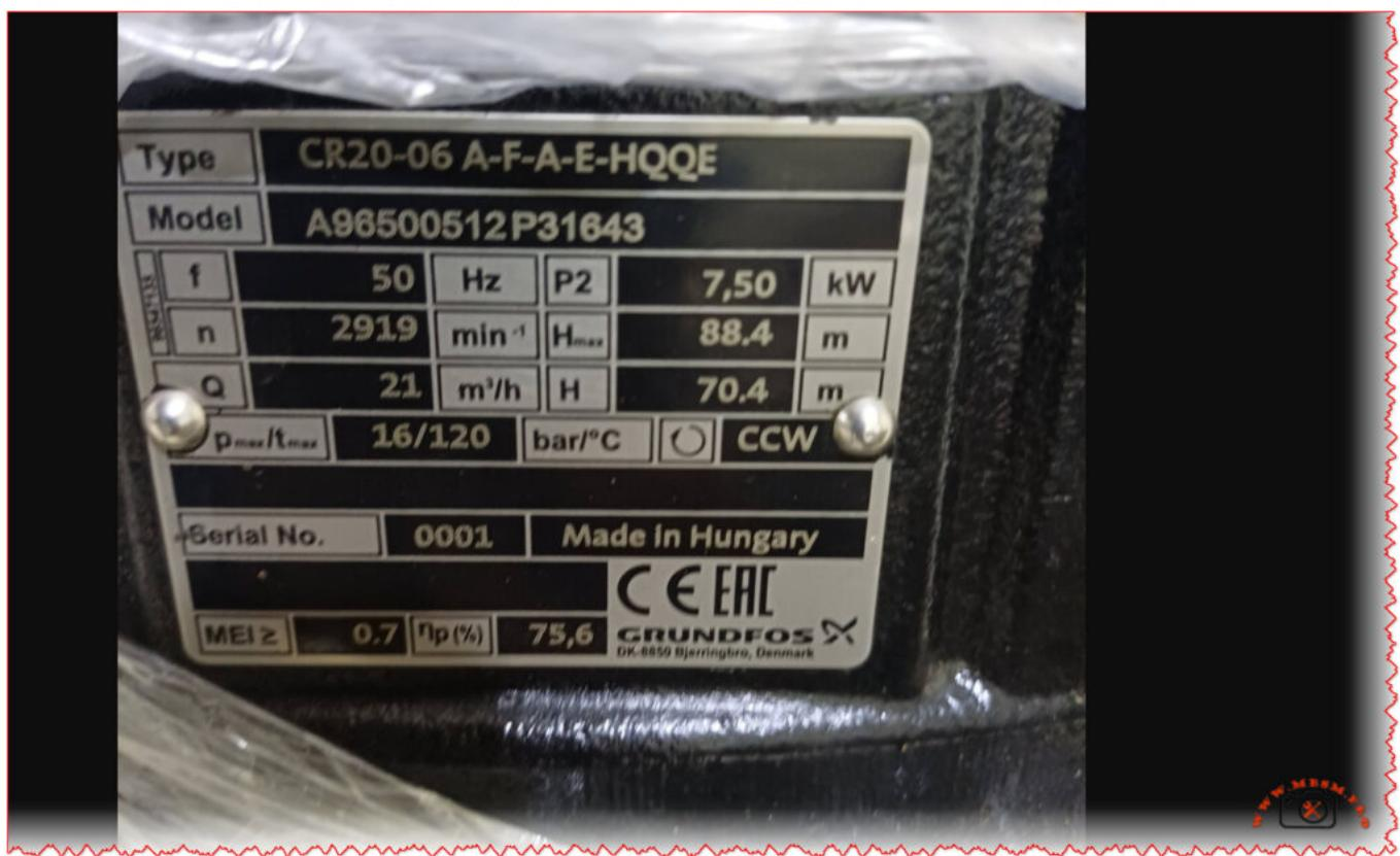
The Grundfos CR20-06 A-F-A-E-HQQE is a vertical multistage centrifugal pump delivering 21 m<sup>3</sup>/h at 70.4 m head with a 7.5 kW IE3 motor, designed for demanding water boosting and industrial applications.
