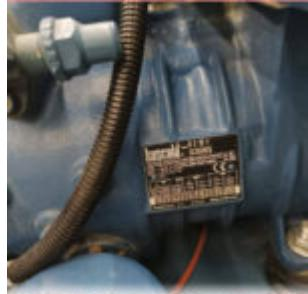
The Frascold D2 15Y is a semi-hermetic reciprocating compressor designed for commercial and industrial refrigeration. With a 2 HP motor and 15.4 m<sup>3</sup>/h displacement, it delivers around 6-7 kW of cooling capacity using R404A, R448A or R449A, making it a robust option for low and medium temperature applications.
