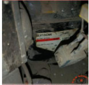
The Danfoss SLV15CNK is a sophisticated variable-speed compressor running on natural refrigerant R290. Designed for commercial freezing applications from -40°C to -10°C, this 15.28 cm<sup>3</sup> inverter compressor requires a dedicated SLV controller and delivers 393-858W cooling capacity depending on operating speed and temperature conditions.
