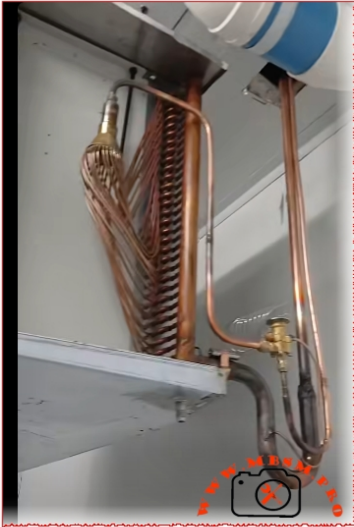
evaporator-cold-room-unit-installation-done-g5 mbsmpro
