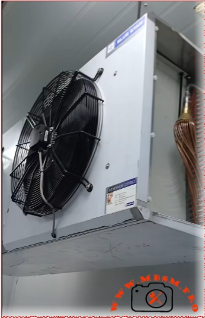
evaporator-cold-room-unit-installation-done-g4 mbsmpro
