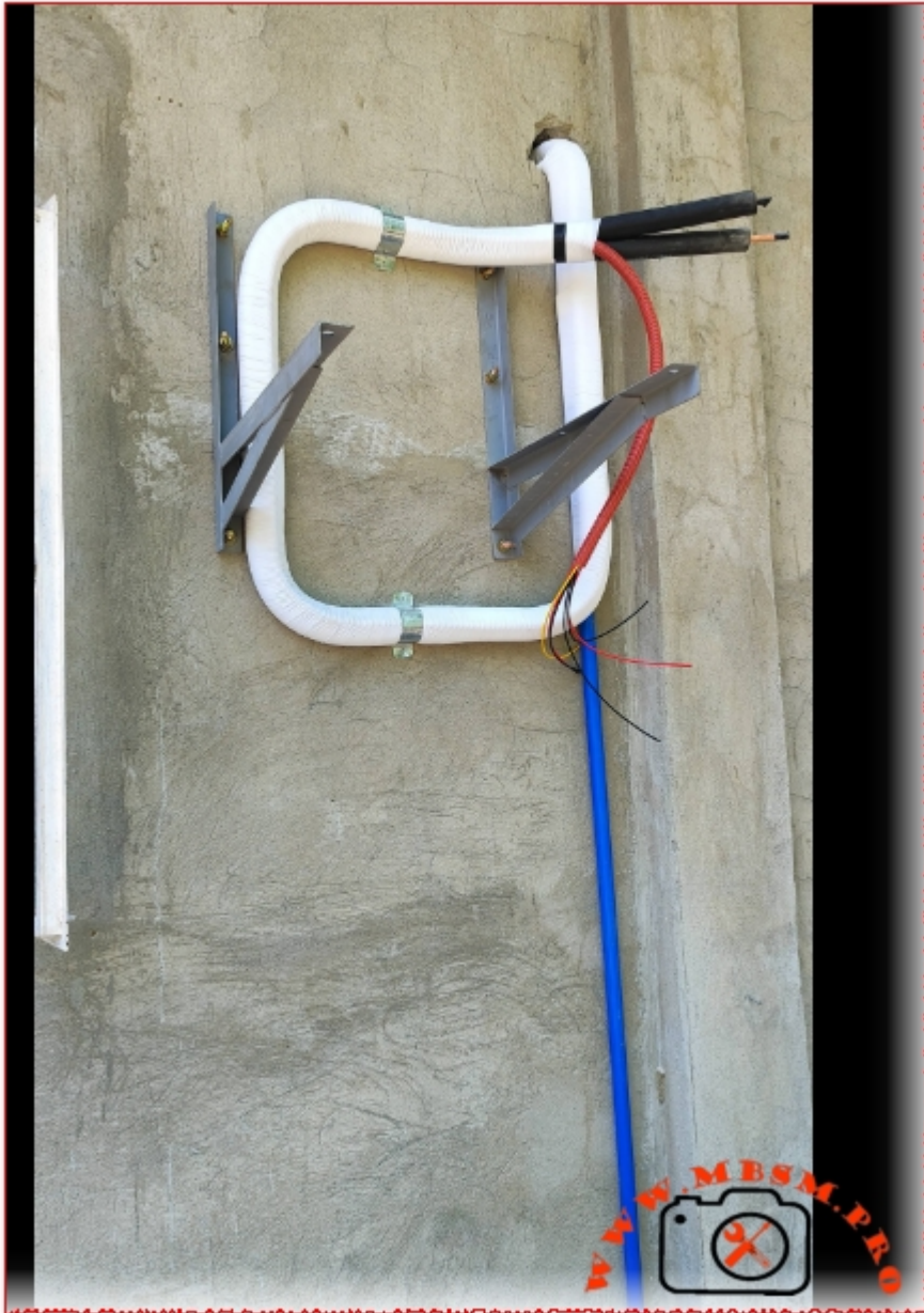
Hisense inverter expert, installtion mbsmpro
