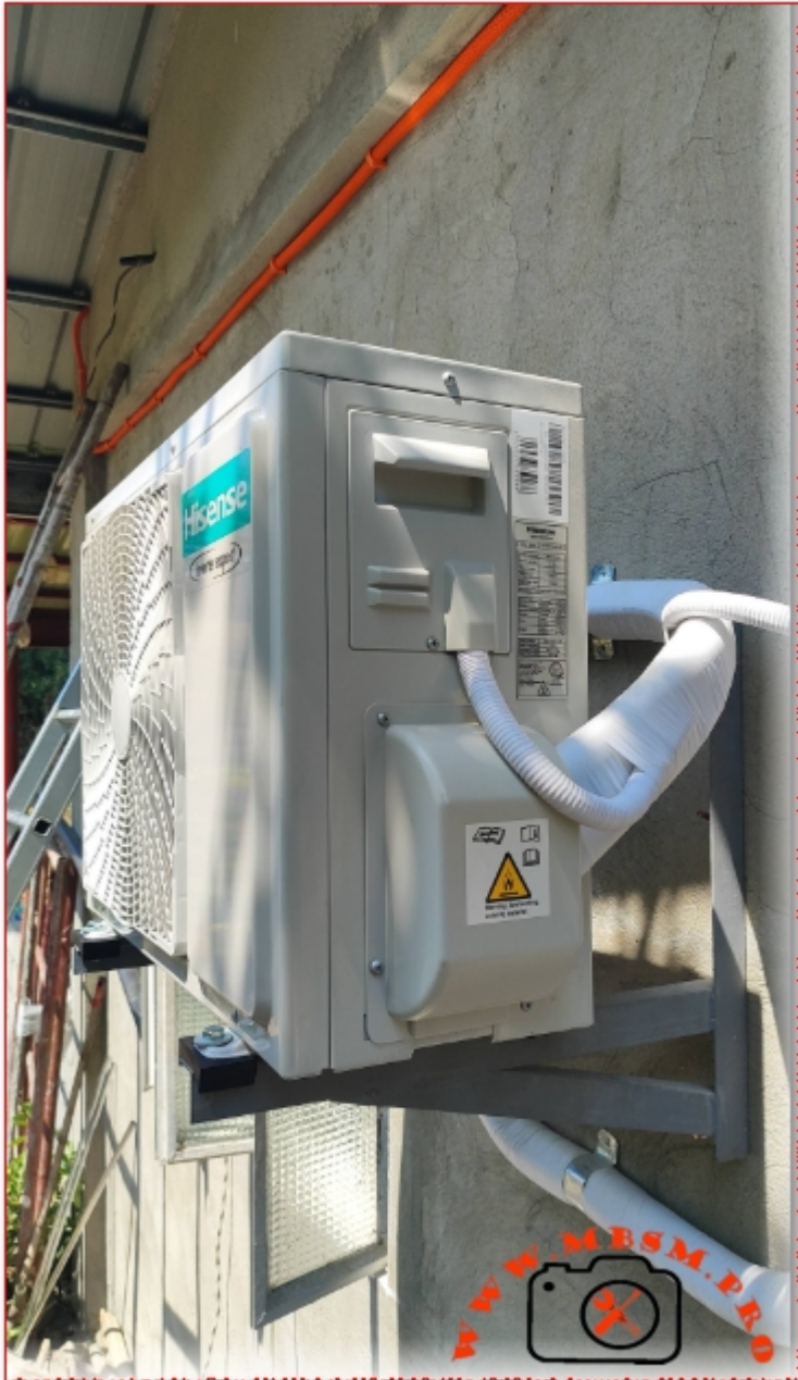
Hisense inverter expert, installtion mbsmpro
