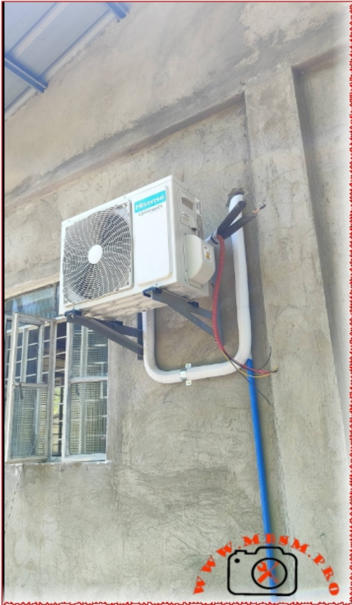
Hisense inverter expert, installtion mbsmpro
