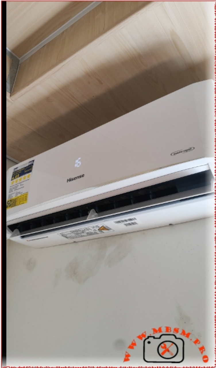
Hisense inverter expert, installtion mbsmpro
