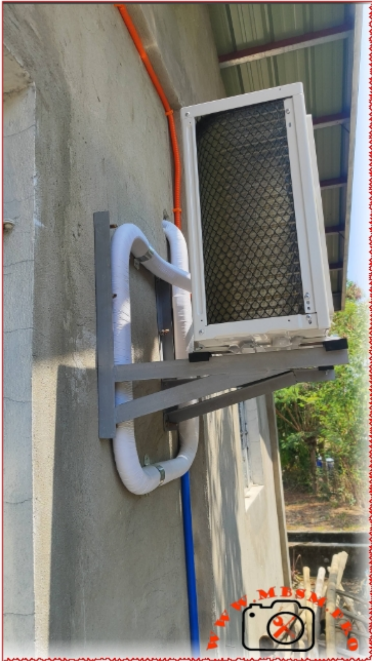
Hisense inverter expert, installtion mbsmpro
