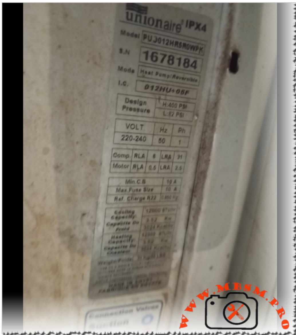
Unionaire PUJ012HR5R0WPK 12000 BTU Heat Pump R22 Technical Specifications and Compressor Replacement Guide mbsmpro
