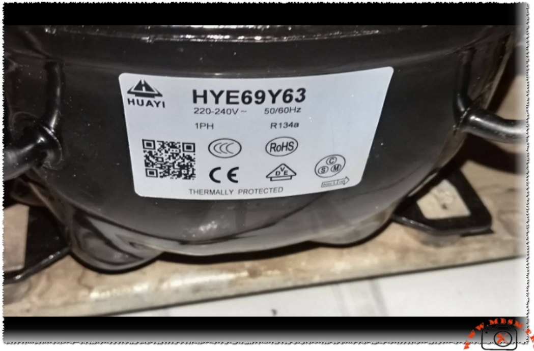
Huayi HYE69Y63 Compressor 1/5 HP R134a LBP mbsmpro
