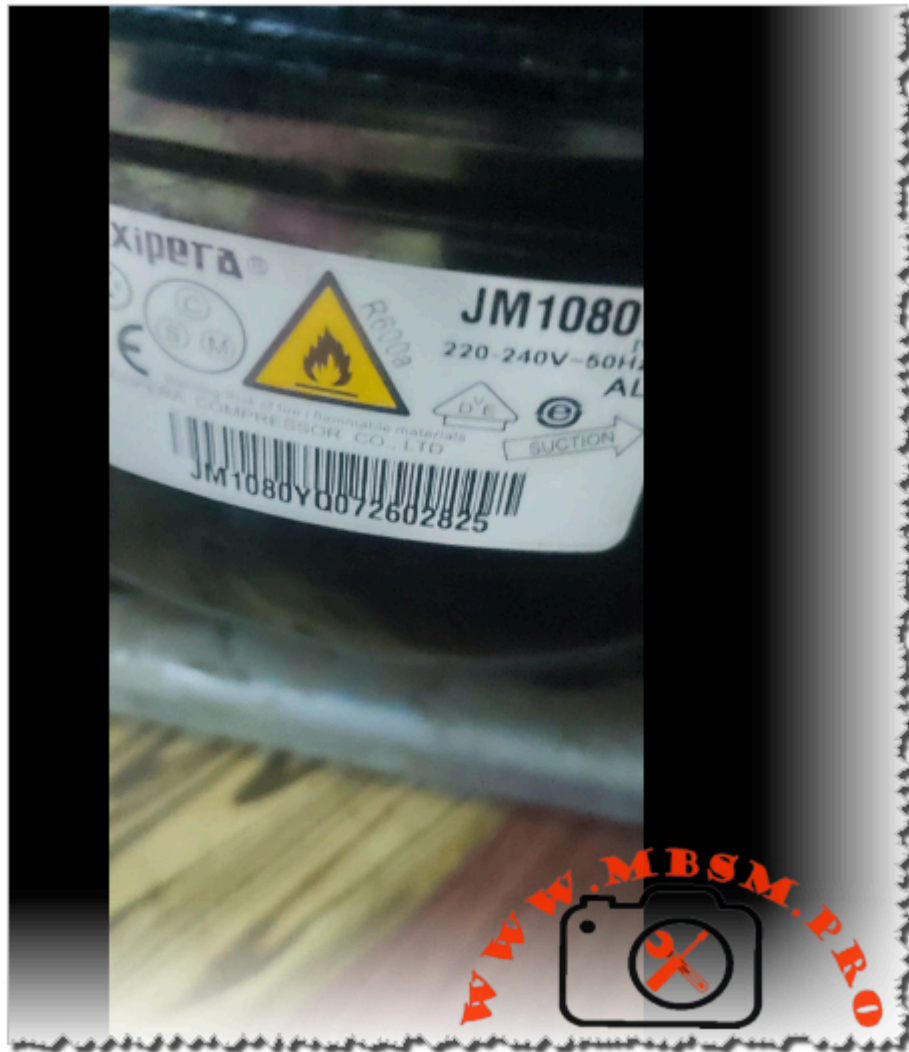
Jiaxipera JM1080y, 1/6 hp+, 143w, r600a, capillary 0.028 inch diameter with a length of 2.5 meters mbsmpro
