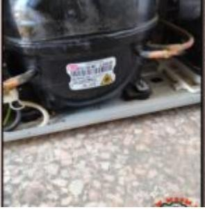
TEE STU 120 MT U252-00 is a hermetic reciprocating compressor from Türk Elektrik designed for domestic refrigerators using R600a refrigerant at low back pressure. It operates on 220-240 V, 50 Hz single-phase supply and delivers around 1/6 hp class cooling capacity, ideal for compact fridges and small freezers.
