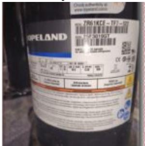
The data plate on the Copeland ZR61KCE-TF7-522 compressor matches the official Copeland Scroll specifications for R407C air-conditioning duty and includes the Copeland authenticity label linking to [copeland.com/v](http://copeland.com/v), a key anti-counterfeit feature. When purchased through an authorized distributor, these details strongly indicate that the unit installed in your system is genuine.
