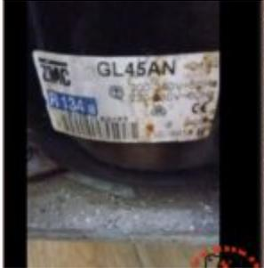
The ZMC GL45AN is a hermetic refrigeration compressor designed for R134a systems in cooling and light freezing applications. With a 1/8 HP motor, LBP operation, and RSIR electrical design, it delivers stable performance, low noise, and high reliability for domestic and light commercial refrigeration equipment.
