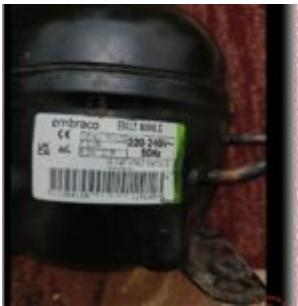
The Embraco EM2Z 80HL.C is a robust hermetic reciprocating compressor engineered for refrigeration efficiency. Featuring a 1/4 HP motor and optimized for R134a refrigerant, this Brazilian-made unit delivers reliable Low Back Pressure (LBP) performance. This guide details its 150ml oil charge, electrical specs, and competitive advantages for technicians.
