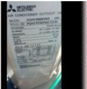
The Mitsubishi Electric PUHY-P250YKH-TH stands out as a powerful 25HP outdoor unit in the City Multi VRF series, designed for large-scale commercial HVAC applications. Featuring R410A refrigerant, it delivers 22.4 kW nominal cooling and 25.0 kW heating capacity with top-tier efficiency.
