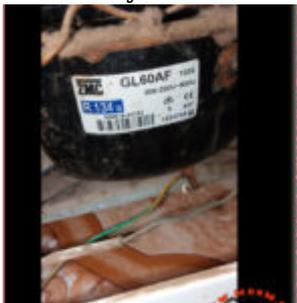
The ZMC GL60AF is a reliable 1/6 HP hermetic compressor designed for R134a LBP applications, widely used in domestic refrigerators and freezers. This comprehensive guide provides complete technical specifications including 5.99 cm<sup>3</sup> displacement, ISO VG 19 ester oil requirements, 132W cooling capacity, and detailed performance data. Find the best replacement options including Cubigel GL60AA, ZEM equivalents, and modern alternatives for your refrigeration repair needs.
