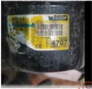
The Secop ES7FT.4 is a high-efficiency 1/5 HP hermetic compressor engineered for R134a LBP applications. With a displacement of 5.70 cm<sup>3</sup> and a cooling capacity of 147W at -23.3°C, it is an ideal choice for tropical refrigeration. This guide provides full technical data, COP metrics, and professional replacement cross-references for HVAC technicians.
