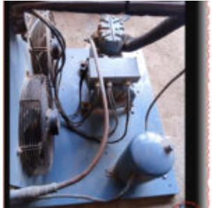
The photos show a Copeland condensing unit on a steel base, with a semi-hermetic compressor, air-cooled condenser and vertical liquid receiver designed for cold room applications. This type of refrigeration unit is widely used in commercial food storage because it delivers stable temperature control, good energy efficiency and straightforward maintenance for professional technicians.
