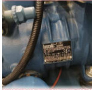
The Frascold D2 15Y is a semi-hermetic reciprocating compressor designed for commercial and industrial refrigeration. With a 2 HP motor and 15.4 m<sup>3</sup>/h displacement, it delivers around 6-7 kW of cooling capacity using R404A, R448A or R449A, making it a robust option for low and medium temperature applications.
