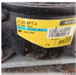
The Secop TLES6FT.3 is a high-efficiency hermetic reciprocating compressor designed specifically for Low Back Pressure (LBP) applications. Operating on R134a refrigerant, this 1/6 HP powerhouse is a staple in domestic refrigeration. This guide breaks down its technical performance, electrical characteristics, and provides reliable replacement options for field workers and engineers looking for precision.
