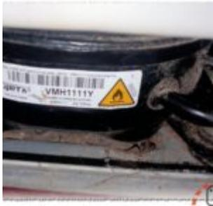
The Jiaxipera VMH1111Y is a high-efficiency variable-speed inverter compressor optimized for R600a refrigerant. Operating between 22Hz and 75Hz, it offers a 1/5 HP equivalent output, making it the preferred choice for premium Sharp and Toshiba refrigerators. This guide breaks down its electrical characteristics, COP efficiency metrics, and professional field-tested replacement alternatives for modern cooling systems.
