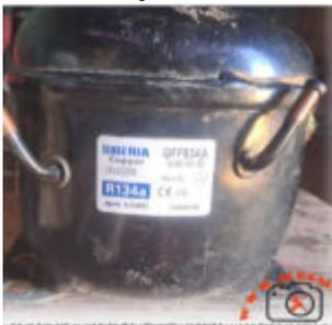
The heart of any reliable industrial or home refrigerator is the compressor. The Siberia GFF93AA stands out as a high-displacement 1/3+ HP unit featuring genuine copper windings and a massive wide-voltage tolerance from 160V to 260V. For technicians working in harsh power zones, this R134a unit provides 270W of efficient, stable cooling power...
