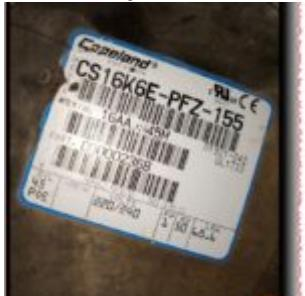
The Copeland CS16K6E-PFZ-155 is a high-efficiency hermetic reciprocating compressor designed for commercial refrigeration. Operating at 220-240V and 50Hz, this 1.25 HP powerhouse is optimized for R404A and R507 refrigerants. Known for its durability in medium-temperature applications, it features POE oil and thermal protection, making it a reliable choice for cold rooms and professional cooling systems.
