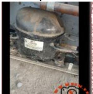
The LG NS24LAEG is a compact 1/12 HP compressor built for R134a LBP systems. You'll usually find this unit running small water dispensers and mini-fridges. Here is the raw technical data and field replacements.
