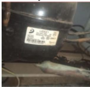
The Donper L65CZ1 is a reliable 1/5 HP compressor designed for R134a LBP systems, commonly found in domestic refrigerators and freezers up to 280L capacity. This guide provides the full technical data sheet, including cooling capacity (158-170W at ASHRAE), oil requirements (280-320ml), and a comprehensive list of compatible replacements for both R134a and modern alternative refrigerants to ensure your repair is successful.
