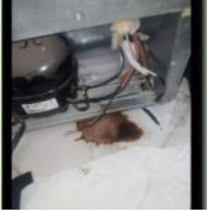
Our technical investigation revealed a dual issue. The system was suffering from a **restricted filter drier**, causing a blockage that choked the cooling cycle. This strain had also compromised the motor's starting components.
