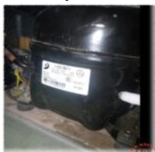
The Donper LG83WZ1 stands as a cornerstone in modern domestic and light commercial refrigeration. Engineered for Low Back Pressure applications, this R134a-driven unit provides reliable cooling capacity for medium to large refrigerators. Its 8.3cc displacement ensures
