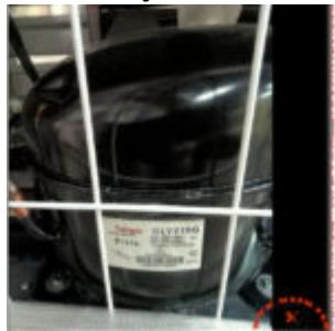
The Cubigel GLY21RG is a robust 5/8 HP commercial compressor designed for R134a systems. Operating in the MBP/HBP range with a 20.72 cc displacement, it offers high cooling capacity for display cases and reach-in coolers. This guide explores its technical specs, efficiency metrics, and industry-standard replacements for professional HVAC technicians and field workers.
