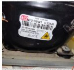
The TEE NTU 170 MT is a high-efficiency hermetic reciprocating compressor designed for low back pressure applications using R600a refrigerant. Known for its reliability in household refrigeration, this unit operates at 220-240V 50Hz. This article explores its technical specs, cooling capacity, and suitable replacements for HVAC technicians and engineers worldwide.
