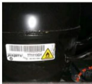
The Jaxipera TT1113GY is a high-performance hermetic compressor engineered for Low Back Pressure applications using R600a (Isobutane). Featuring a 11.3 cm<sup>3</sup> displacement and a cooling capacity of 183 Watts, it represents the gold standard for modern energy-efficient refrigeration, offering exceptional reliability and reduced acoustic emissions in the domestic market.
