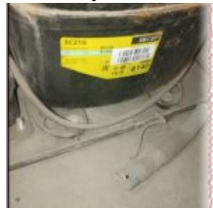
Secop SC21G is a high-performance hermetic reciprocating compressor designed for commercial refrigeration and freezing applications using R134a refrigerant. This guide covers detailed specifications, technical parameters, and installation requirements for 220-240V/50Hz systems at up to 1.3 amperes.
